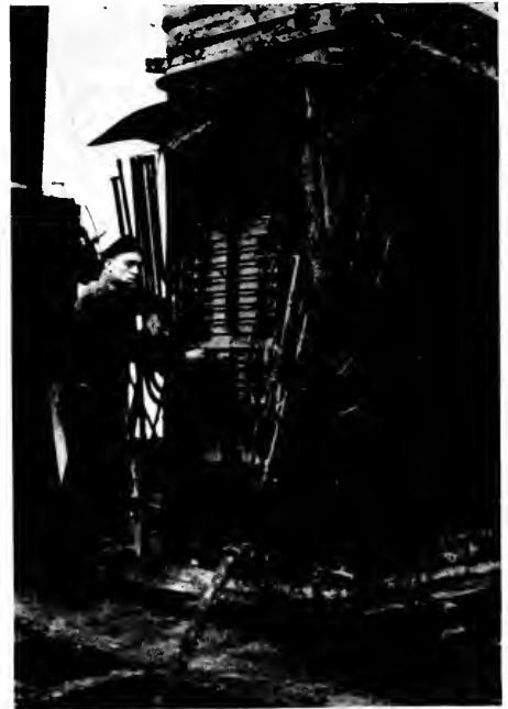
A switchboard on the bridge deck. The armored conduit stood the fire perfectly.
